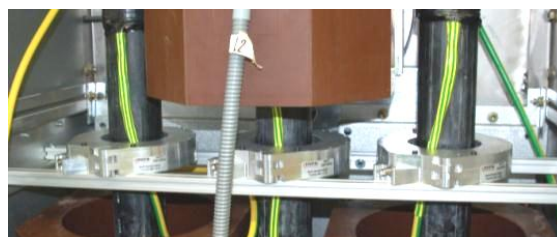
Figure 2 Examples of HFCT sensor attachment
