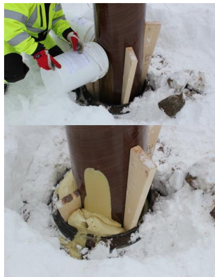
Figure 6 Fixing the pole (Photo: NTE Nett)
