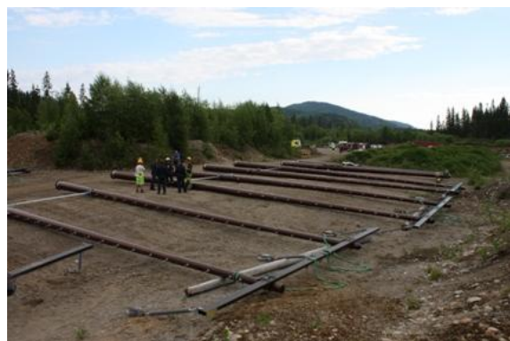
Figure 7 Preassembling of the poles (Photo: NTE Nett)
