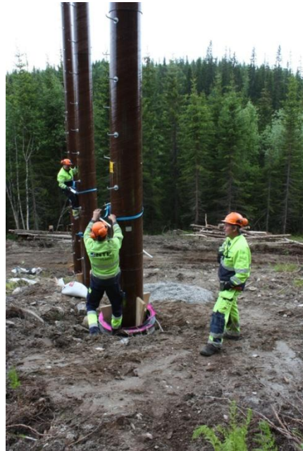
Figure 5 The poles are placed (Photo: NTE Nett)
