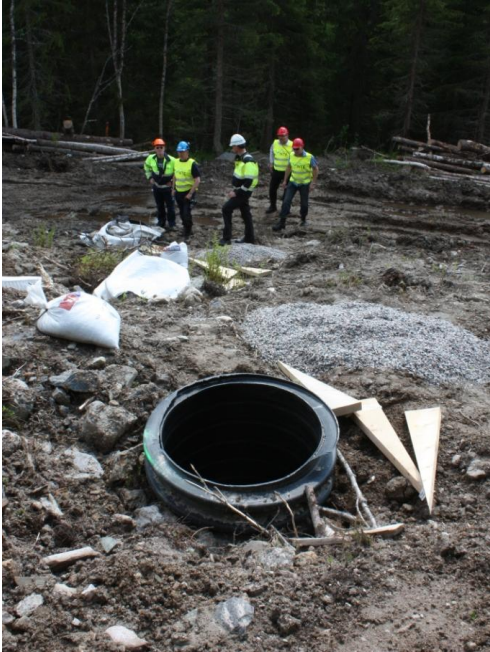
Figure 3 Foundations are ready (Photo: NTE Nett)
