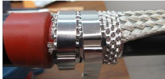
Figure 2-6: Screen connection by a copper braid, "cheese grater" contact plate and cable clamp ('Ligarex').
