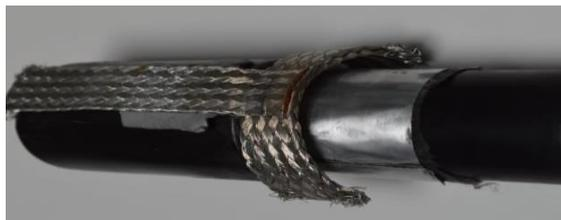
Figure 2-9: Screen connection by a copper braid for a combination with heat or cold shrink tubes.
