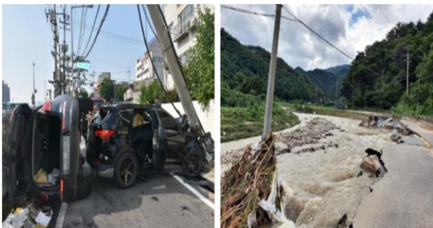
Figure 9: damages on poles detected in real time with tilt- and acceleration sensors, paper 10599.
