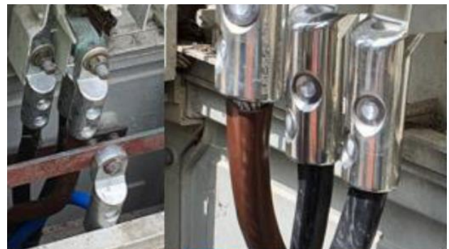
Figure 15: Screw terminals with torque limiter - Paper 11184
