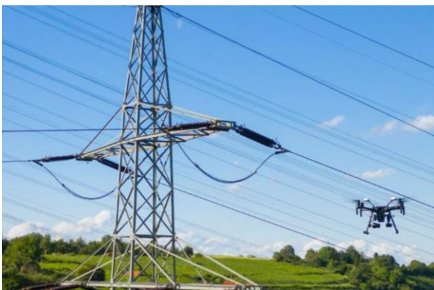
Figure 5: satellite image for vegetation management and use of drones for inspection of lines and poles, paper 10135.
