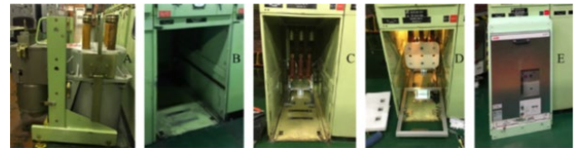
Fig. 4 from paper 0384: Vertical racking bulk-oil circuit-breaker (A) and the retrofit installation steps (B to E).
