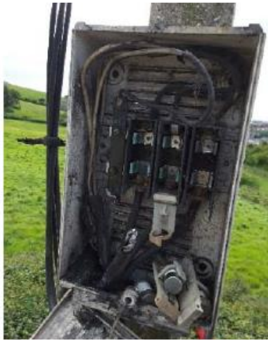
Fig. 40: Neutral loss detected (high priority intervention) (paper 851)
